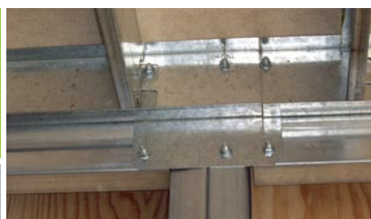
Finished mezzanine floor within a building ready for wall lining
