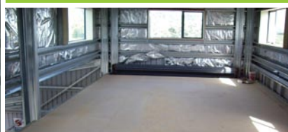
Finished mezzanine floor within a building ready for wall lining
