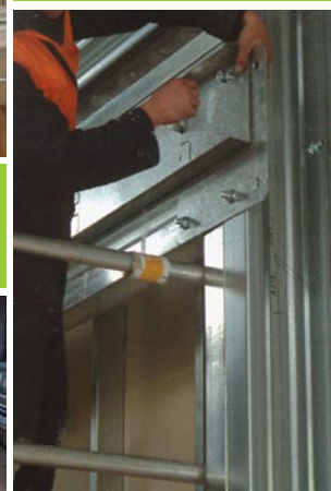
Installation of RFS Perimeter Channel
