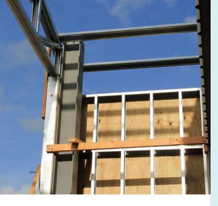
The RFS 150mm Framing replaces its timber equivalent and can be use in a myriad of applications. The 150mm Framing residential applications include high stud walls, mid-floors and roof panels. The 150mm Framing can also be used in the commercial environment, for internal and external walls, inter-tenancy walls and fire-rated walls.
