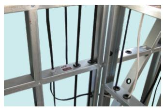
Swaged nogging for easy insertion into stud.
