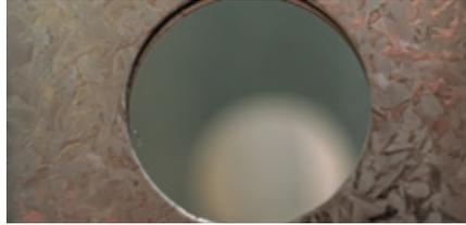
Pre-formed 32mm holes, allow for services to be easily accessed and fed throughout the walls.
